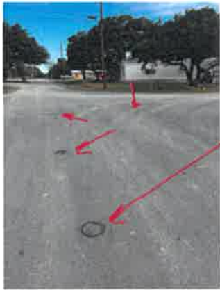
WATER LINES IN MIDDLE OF STREET THESE ARE INLINE VALVES
