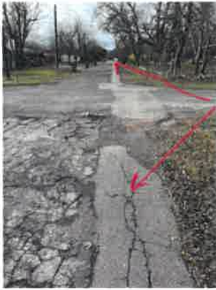
SEWER LINE EXTENDS ALONG STREET SEVERAL VACANT LOTS WILL REQUIRE SIMILAR TAP AS ABOVE
