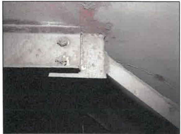
Bull Ring detail. Please note that dimensions shown are for a much larger tank. The dimensions would need to be adjusted accordingly for the Blanco Standpipe.
