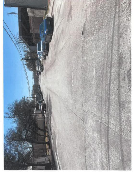
Road surface is relatively smooth, raveling of pavement, some edge deterioration.
