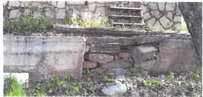
Section 3 is leaning and is cracked. (2018)
