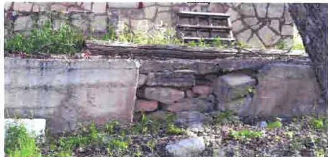
Section 3 is leaning and is cracked. (2018)
